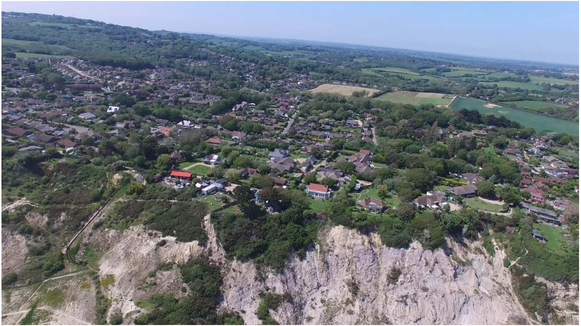
Figure 9.1 Above: View of properties located seaward of Cliffway and Rockmead Road close to the edge of the cliff.
