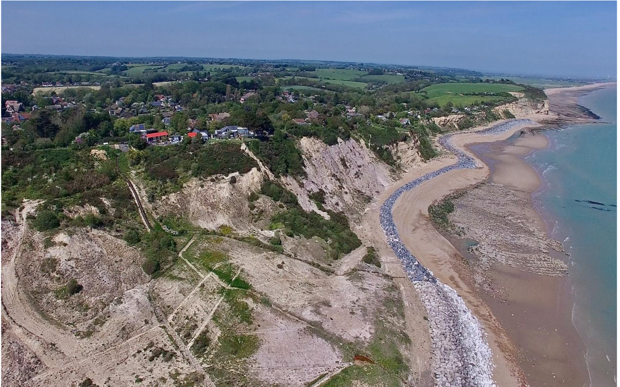
Figure 4.4 (Above) and 4.5 (Below) show the extent of the surface water drainage provided as part of the Phase 2 scheme fronting Rockmead Road. A line of wells and pneumatic pumped drains along the road behind and parallel with the sea cliff assists in lowering groundwater levels.
