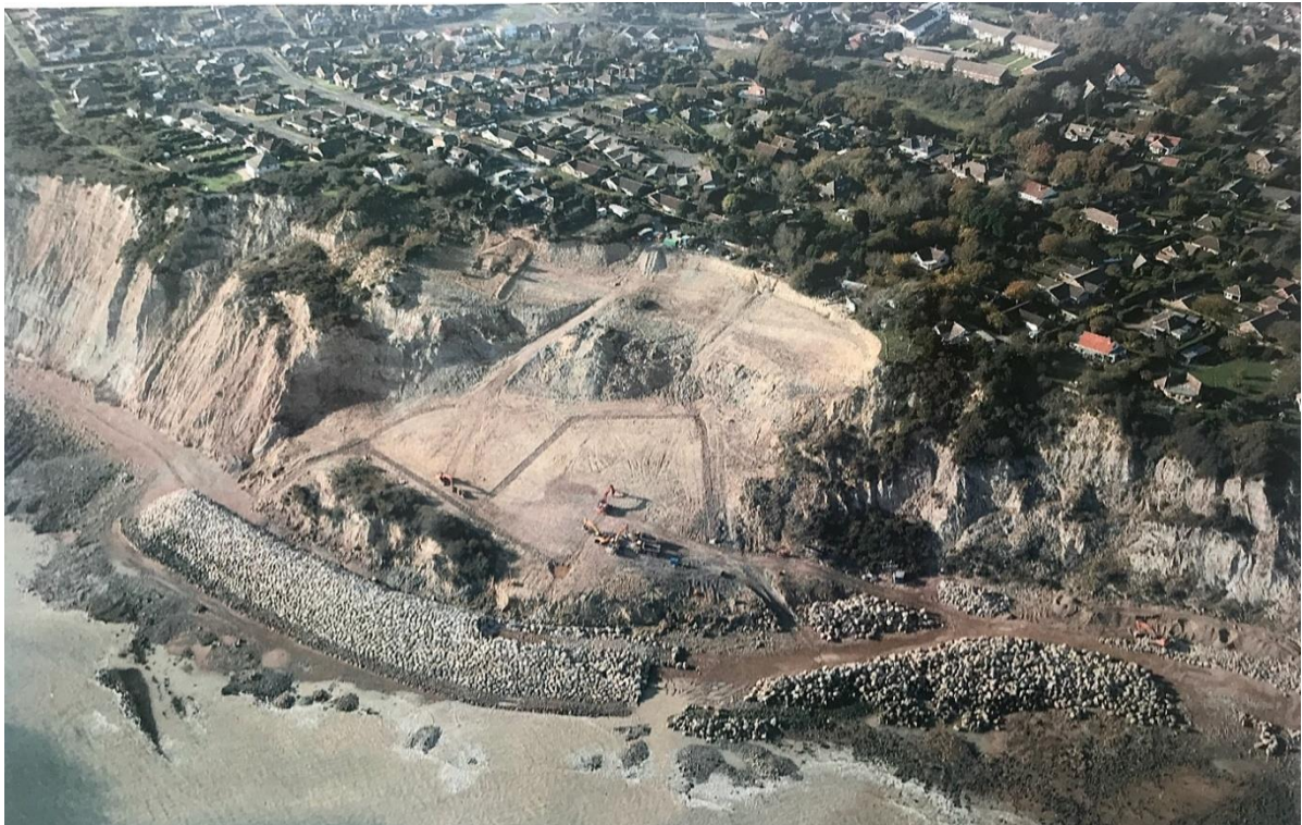
Figures 3.1 (above) and Figure 3.2 (below) showing work in progress on the phase 2 scheme for coast protection and drainage works along the Rockmead Road frontage in 2008. Photos: Prof Roger Moore.
