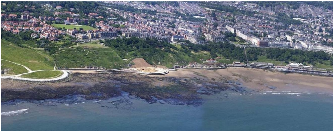
Figure 8.1 (Above) show the Holbeck hall Hotel landslide site at Scarborough following completion of a programme of coastal protection, slope stabilisation and drainage works. Ongoing management is achieved through maintenance, monitoring and engagement with stakeholders. Images courtesy of Scarborough Borough Council.
