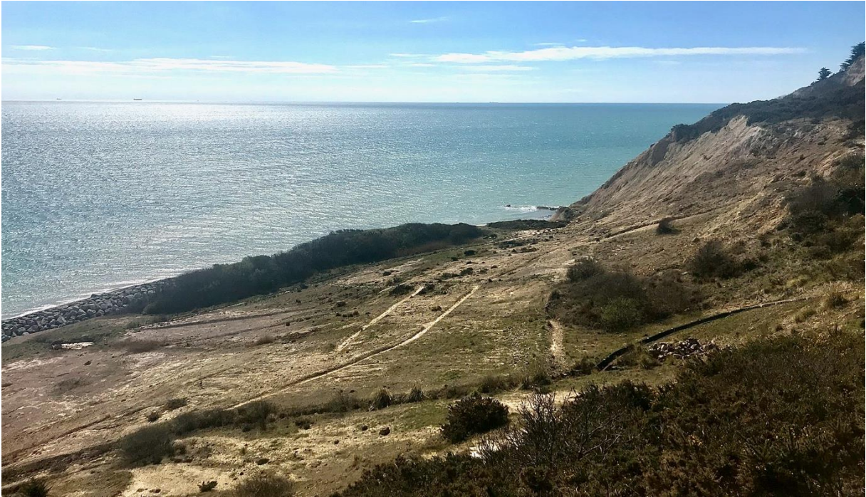
Figures 4.6 Above and 4.7 Below show the coastal slope fronting Rockmead Road and the layout of ditches include the main line ditch, which discharges pumped groundwater flows from the drainage wells down towards the sea.
